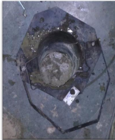
Fig 14. Tamping of concrete
